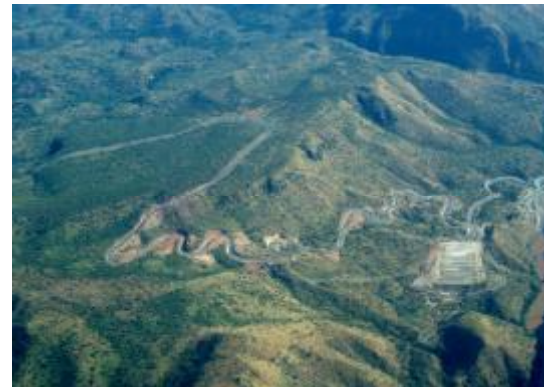
The 420 MW Gibe II Hydro power dam under construction in Ethiopia
